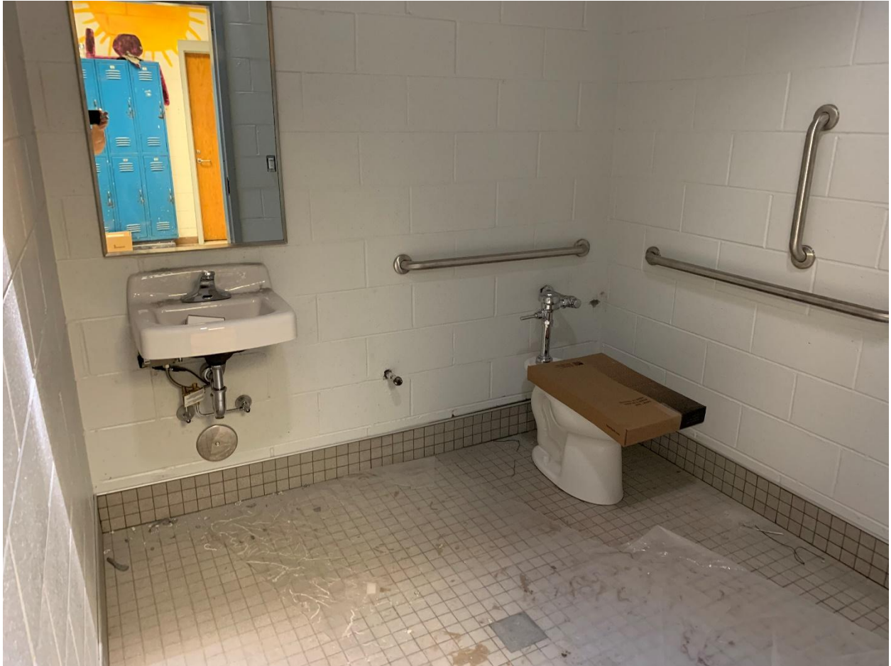
Another handicapped assessable restroom.
